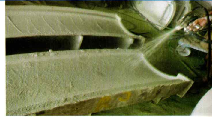
GRC Casting with spray process
